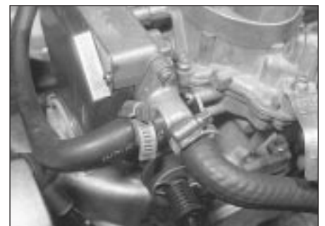
8.5b Coolant hose connections to carburettor auto-choke
