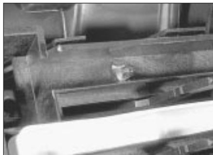
4.14 Heater control panel bulb (arrowed)
