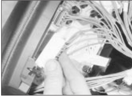
7.17a Instrument panel wiring connectors
