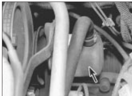
7.3b Hydraulic pump (arrowed)
