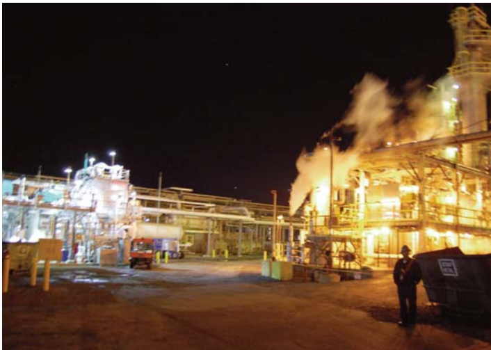
New SafeSite® LED lighting on the left and HPS lighting on the right
