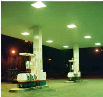
Canopy lighting includes airports, drive-through facilities and gas stations.
