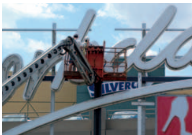
Installation of the LED-System.
