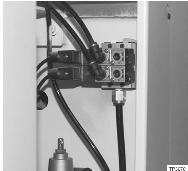
Figure 2.4 - Air Solenoid Valves
